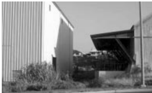
Entrance to warehouse (left bldg) observed from street
