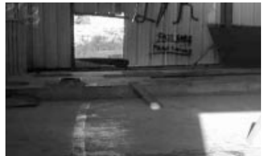
Photo depicts tire marks across floor through hole in wall
