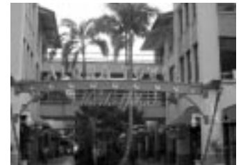
Aloha Tower Marketplace located adjacent to Honolulu Harbor
